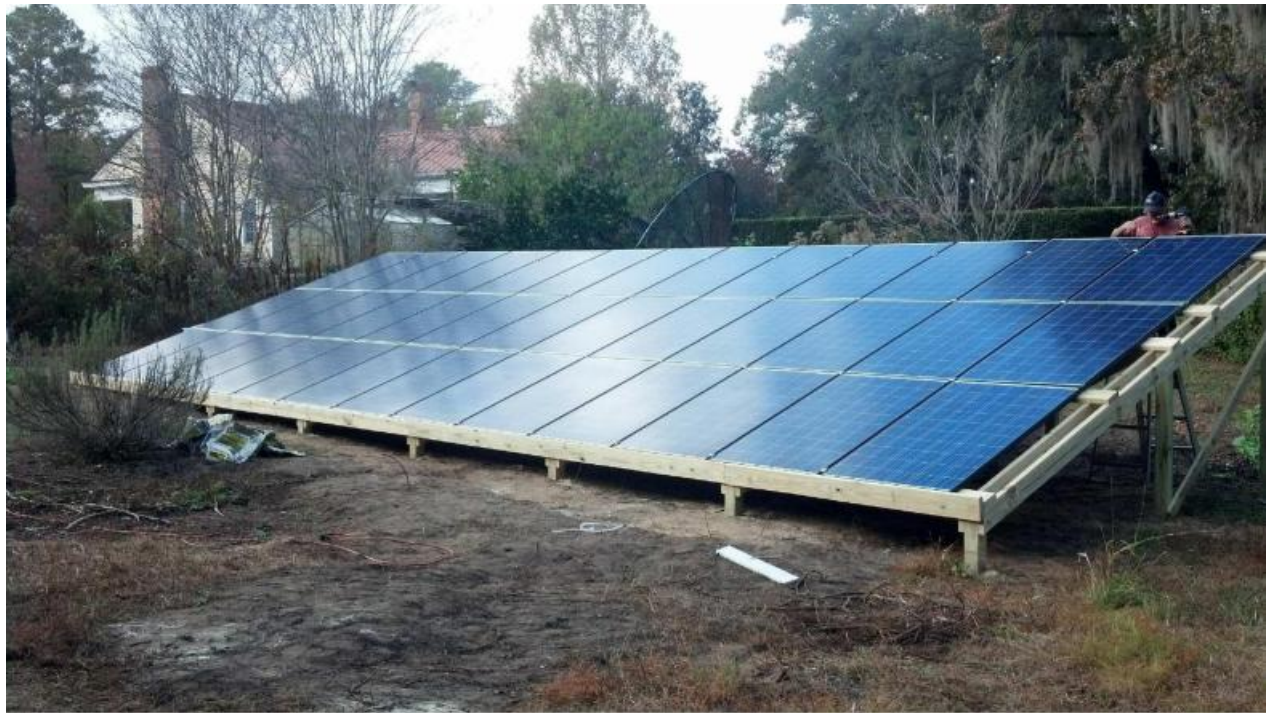
TYPICAL GROUND MOUNT PV ARRAY
